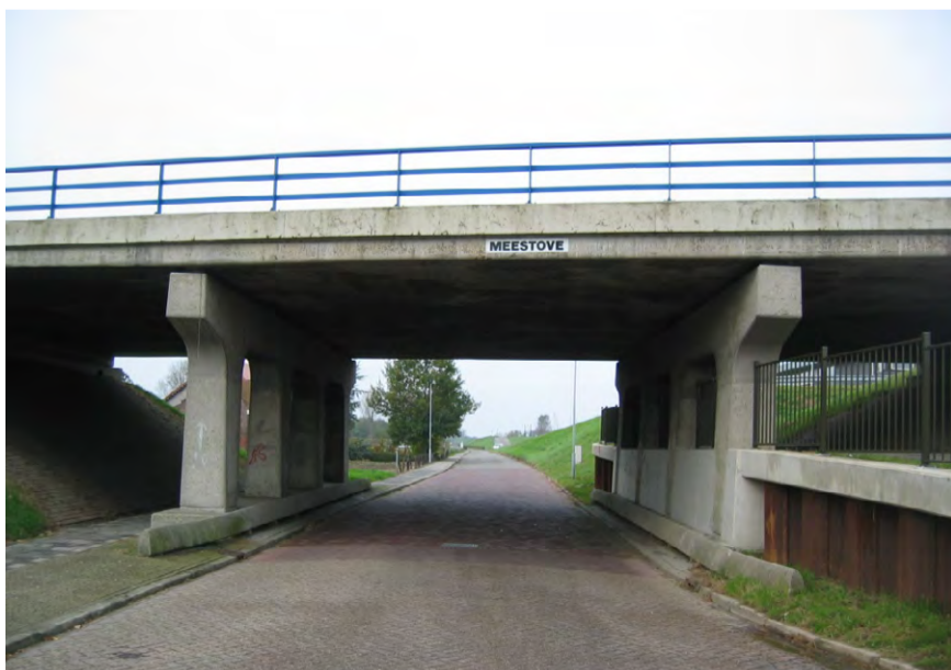
Viaduct N59 - noorddijk
